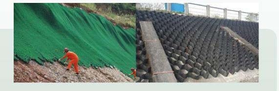
Along the slope the Geocells should be anchored with rebar with BaseCaps typically 12-18" in length depending on the consistency of the slope material. The spacing between the rebar shall be determined by design with each rebar placed on the junctions of the panel.
