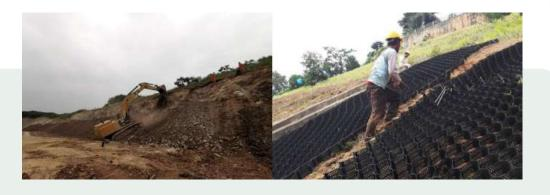
Excavate anchor trench where an anchorage trench is specified, each panel should be anchored at the top of the slope in a trench whose dimensions are determined by design depending on the geometry of the slope. For shallow slopes, anchor trenches may not be required as pins used to fasten the system to the slope can provide sufficient anchorage strength.
