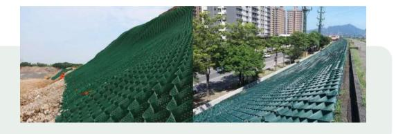
If seeding is specified then it is recommended to place the seeds approximately 3/4" below the finished level. Application of a further 1/2" layer of fine top-soil (such as sandy loam) is recommended after seeding and this final layer should be lightly raked (using the back of the rake) to evenly cover the Geocell cells.
