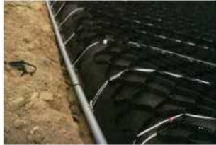
Tendon secured with Pipe
