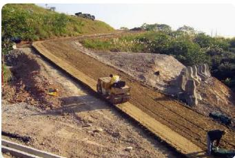
① Once the cells are filled and the system is compacted, the Geocell base is ready to withstand heavy traffic loads.
