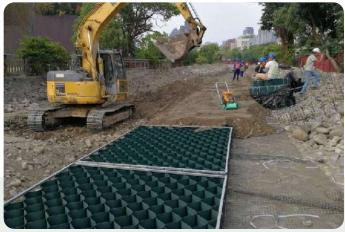
Fill the first rows of cells with a front-end loader or dump truck and push the fill into cells using shovels or abulldozer blade. A 'ramp' of fill material immediately adjacent to the Geocell will likely be necessary to allowequipment to climb onto the system. Continue until all cells are filled. Never allow any equipment to drive overunfilled cells. Always overfill the cells slightly to allow for consolidation.
